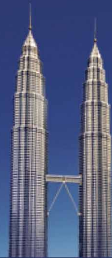
Twin Towers, Malaysia
