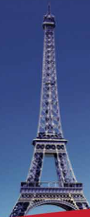
Eiffel Tower, France
