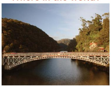
MADE from wrought-iron, this bridge was built in Manchester, England in 1864 and was then shipped halfway across the world to be assembled in its current place.
